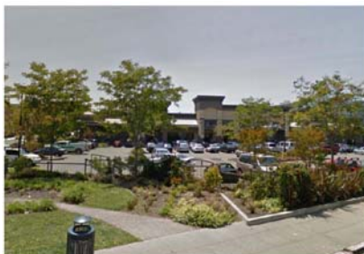
Parking lot—landscaping and relationship to buildings and sidewalks
