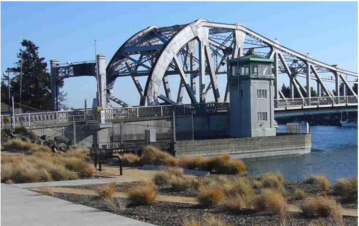
Existing Condition with Catwalk on Fender
